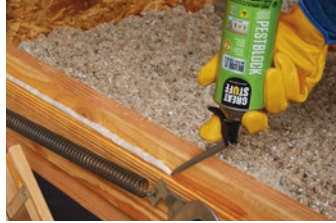
Attic Hatch Frame
