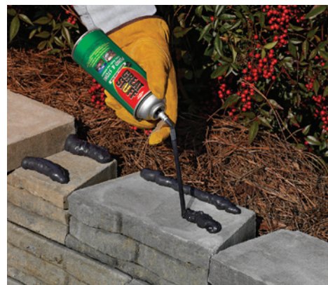
Adhere Cap Stones In Retaining Walls
