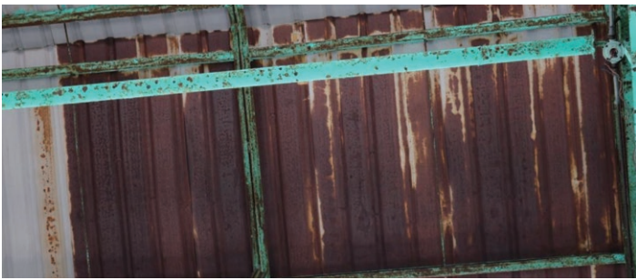
Original steel sheet roofing
