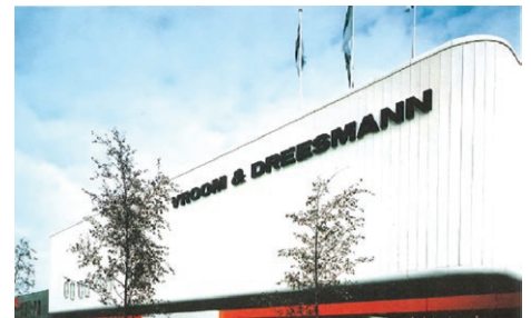
Shopping center (Netherlands)
