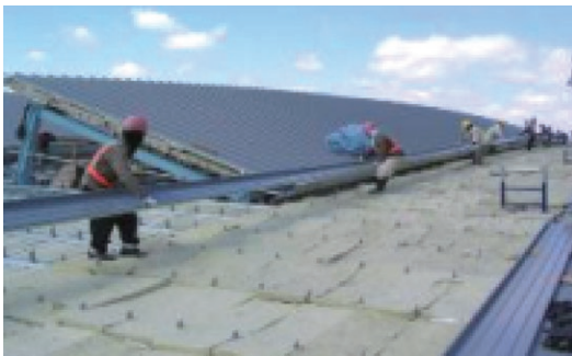
Simultaneous laying of roof panels
