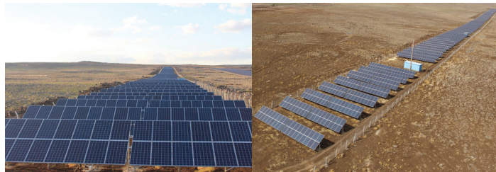
Aerial views of the 1 megawatt solar plant in Kilis, Turkey
