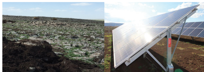
The rocky terrain and the solar panels fixed at an azimuth of 37 degrees to help maximize production
